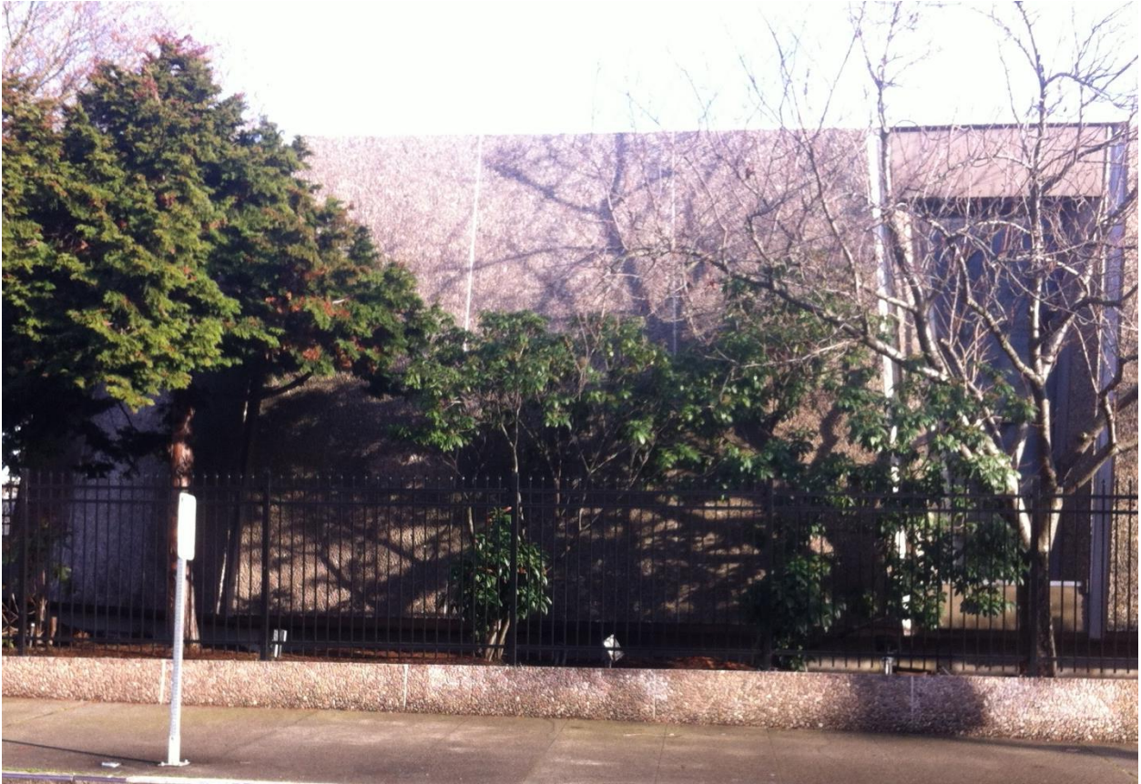
Figure 10: Western elevation looking east. Window panel is part of the 1985 addition which extends to the south. Photo Date: January 6, 2016.
