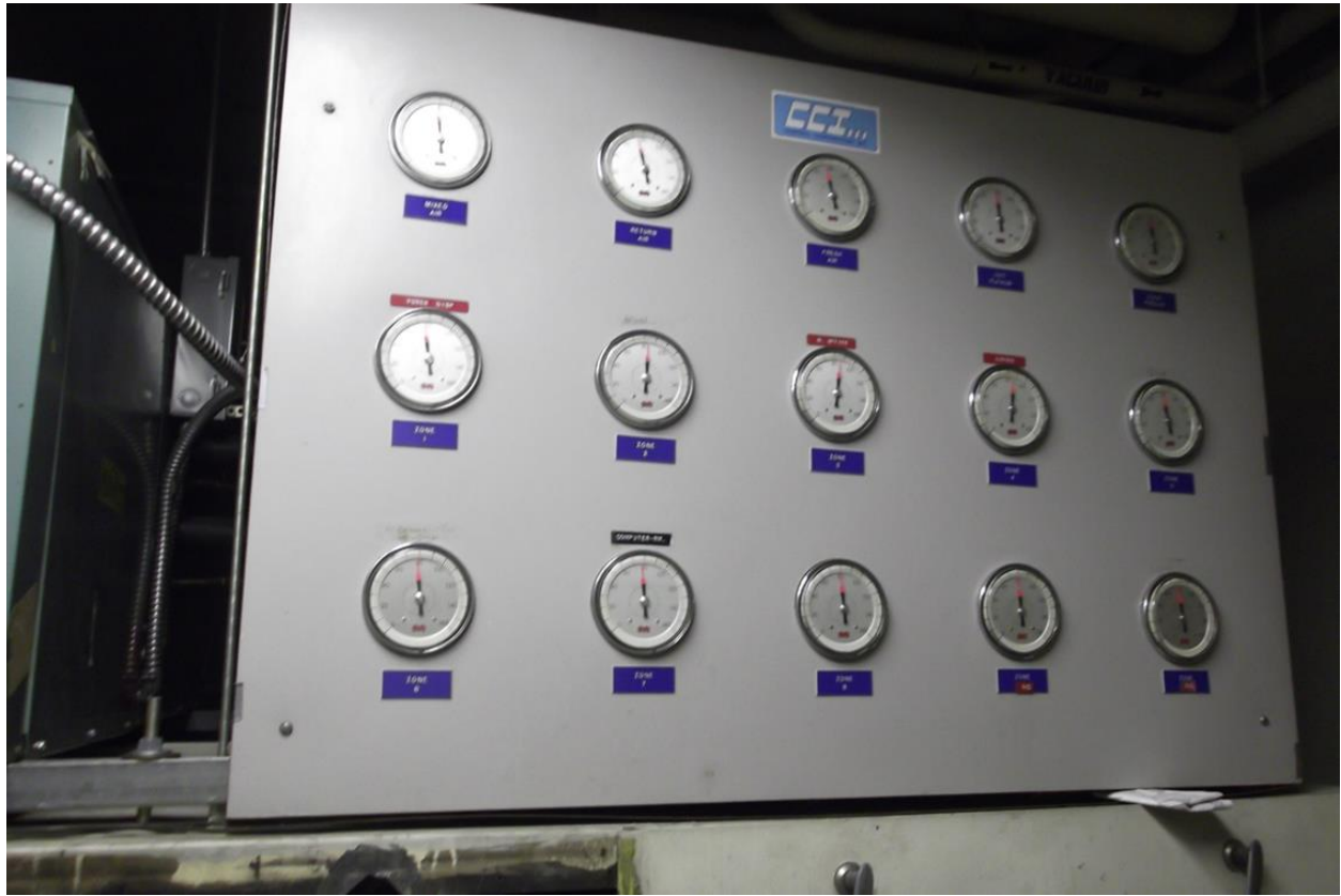
Figure 22: Gauges added in the basement addition of 1985. Photo Date: 2015.
