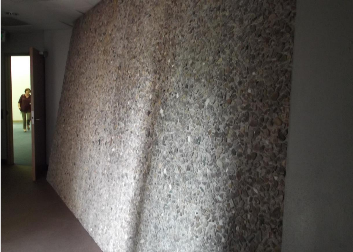
Figure 19: Original exterior wall of southern elevation, looking west. Photo Date: 2015.
