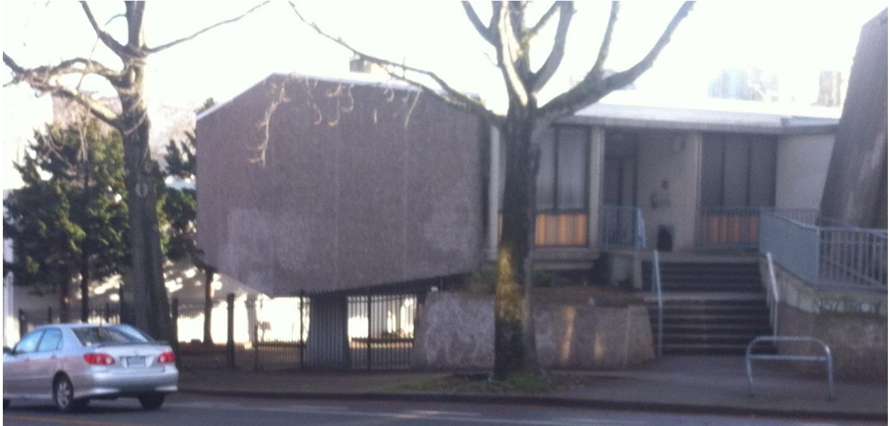
Figure 5: North and west elevations of six-sided office wing looking southeast. Photo Date: January 6, 2016.
