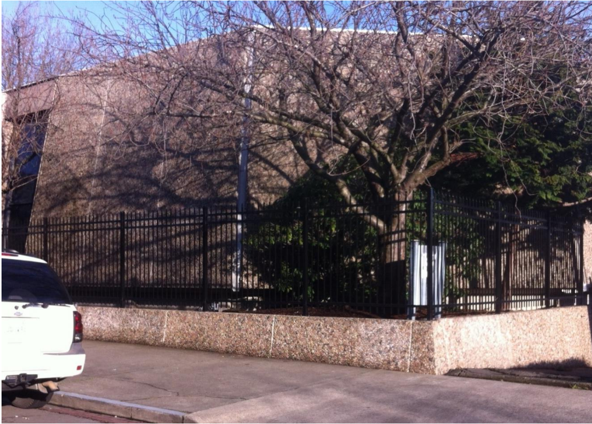
Figure 12: Southwest corner. All panels added in 1985. Photo Date: January 6, 2016.
