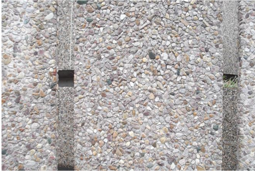
Figure 18: Texture of large polished stone aggregate finish. Photo Date: 2015.
