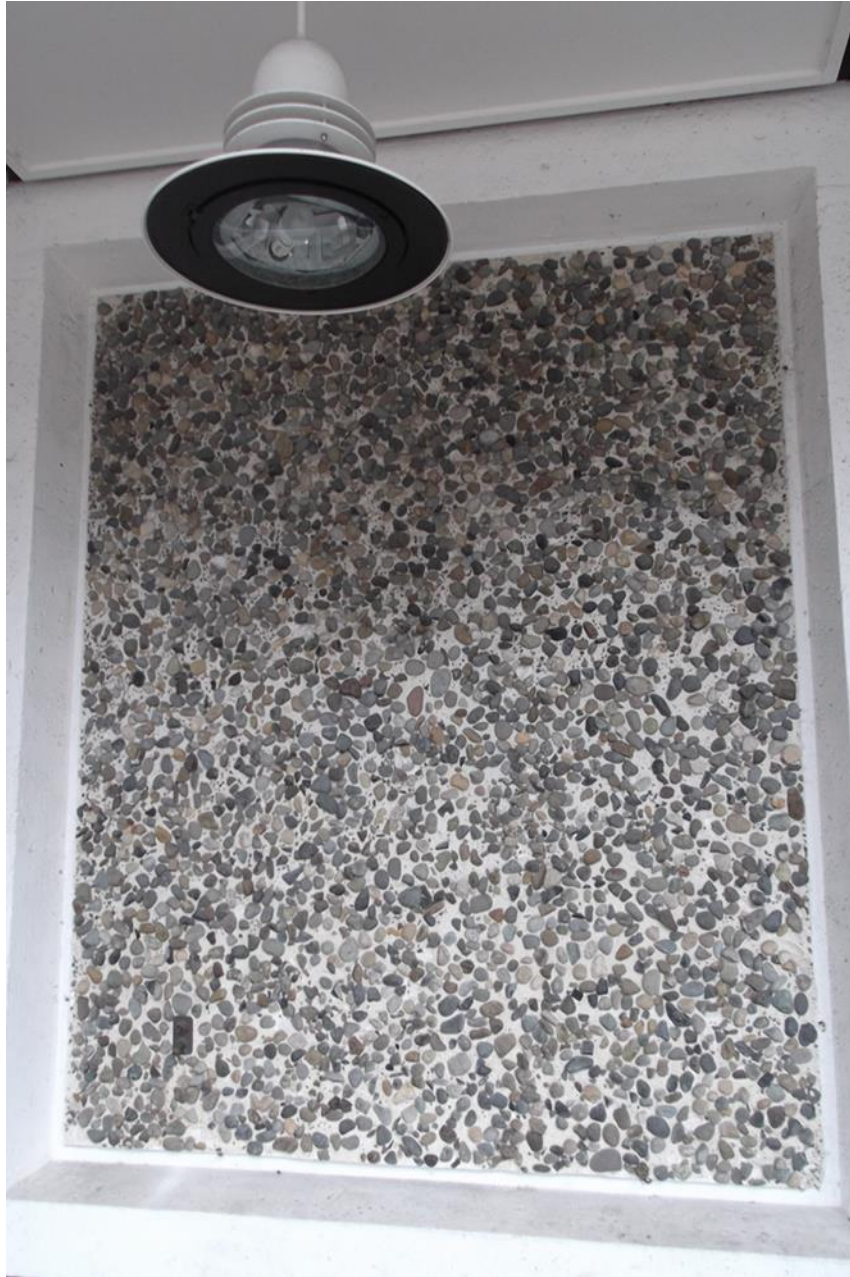
Figure 39: Stone panel and light fixture at offices of Harmon Pray & Detrich. Looking east. Photo Date: 2015.
