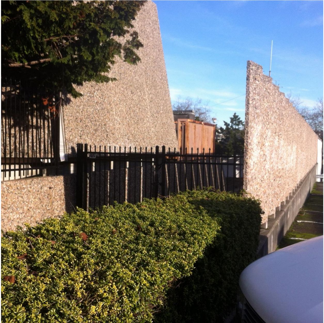
Figure 13: Looking east showing southern elevations and decorative fence. Photo Date: January 6, 2016.
