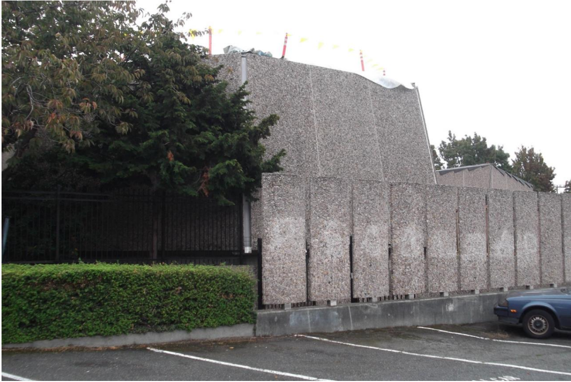
Figure 16: South elevation of 1985 addition with 1963 fence panels. Looking northeast. Photo Date: 2015.
