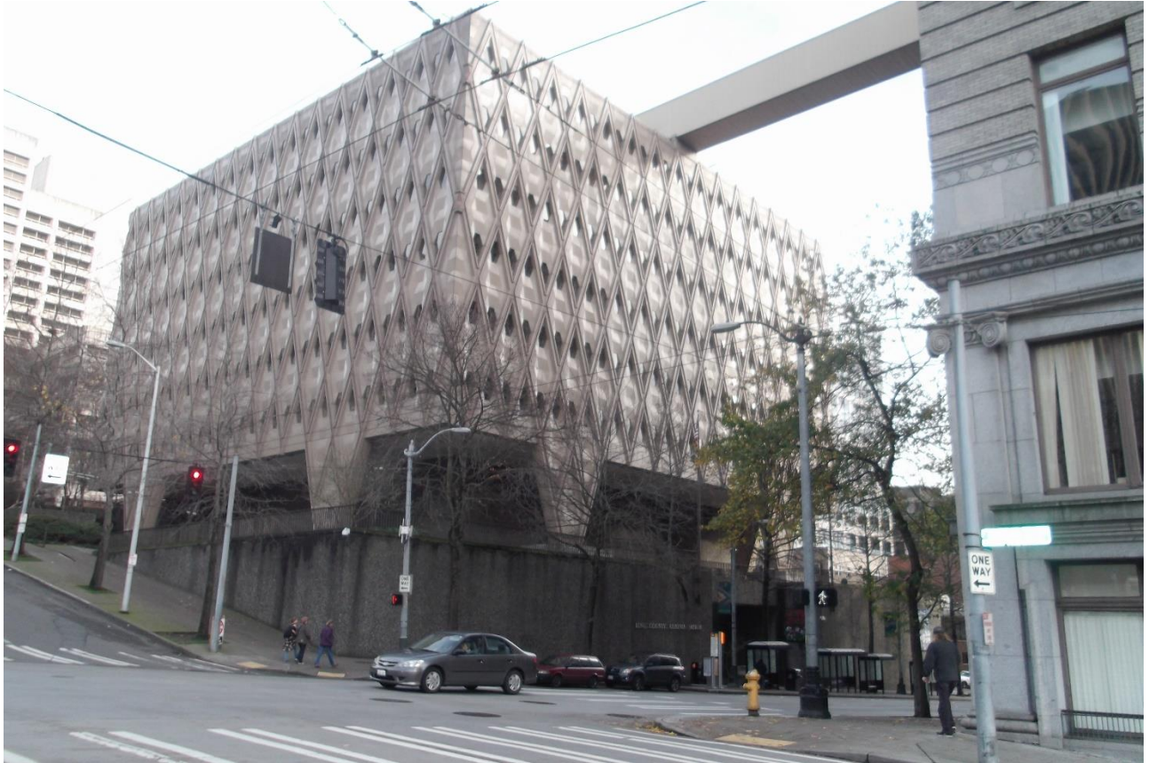
Figure 41: King County Administration Building looking southeast. Photo Date: January 18, 2016
