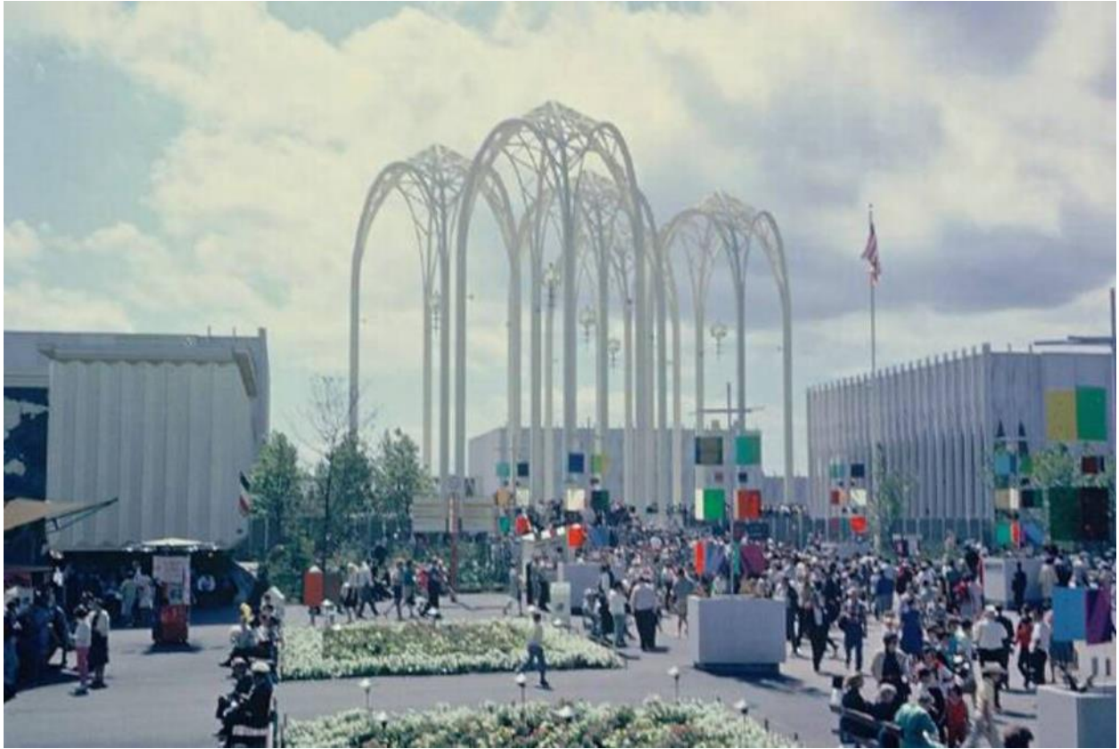
Figure 3: Pacific Science Center. Minoru Yamasaki. 1962. Looking south. Photo Date: 1962.
