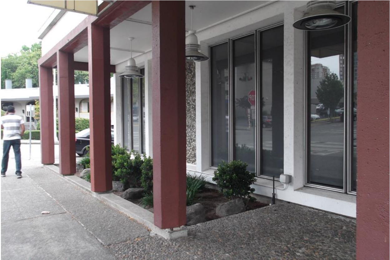
Figure 38: Offices of Harmon Pray & Detrich, 2230 8th Avenue looking north. Photo Date: 2015.
