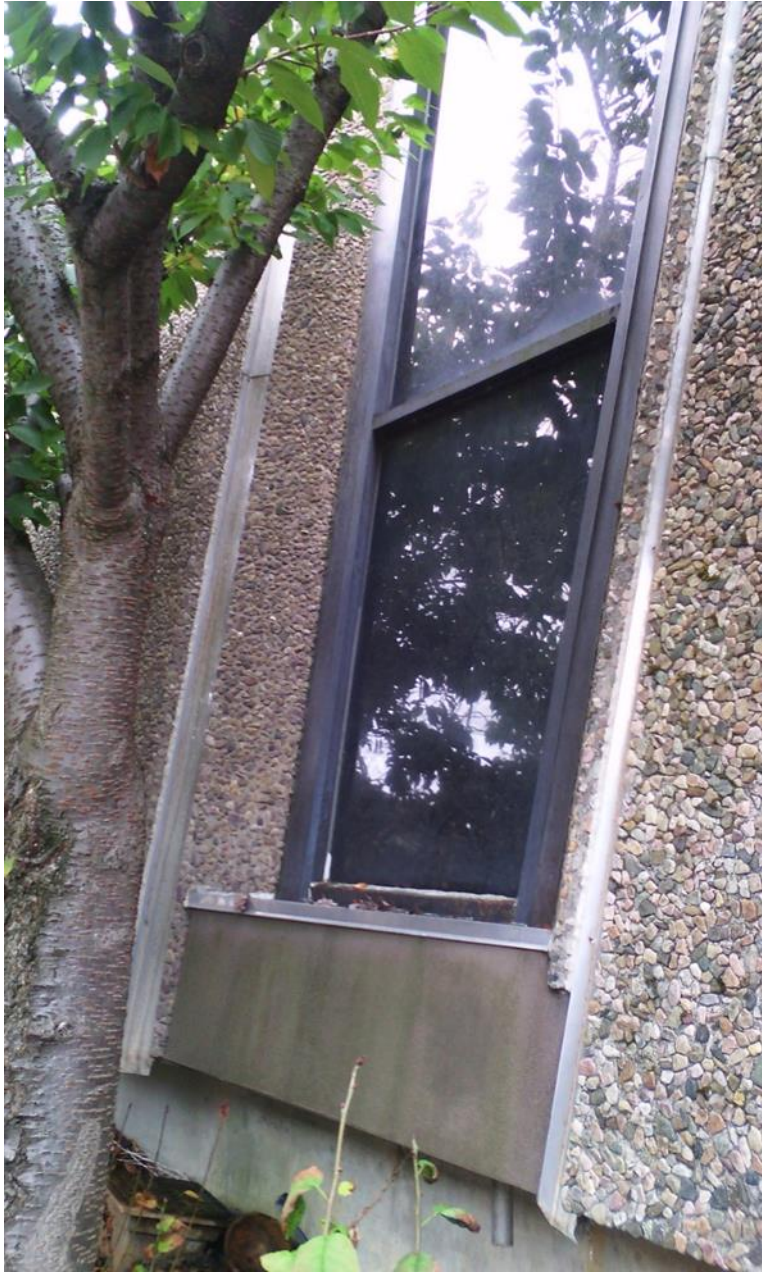
Figure: 20: Western façade looking northeast at 1985 window addition. Photo Date: 2015.
