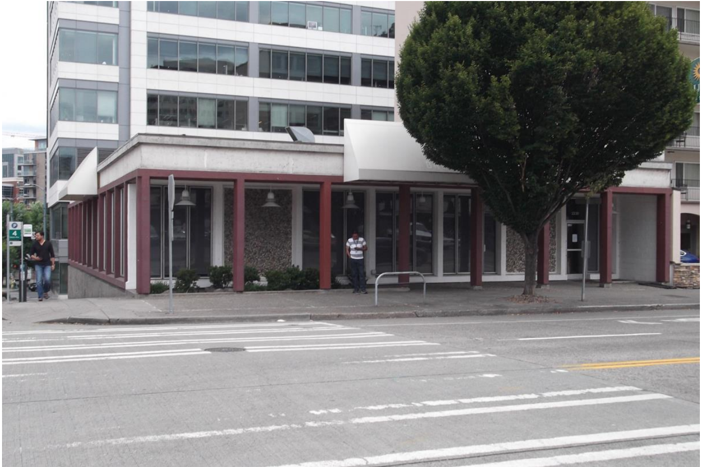
Figure 37: Offices of Harmon Pray & Detrich, 2230 8th Avenue looking east. Photo Date: 2015.
