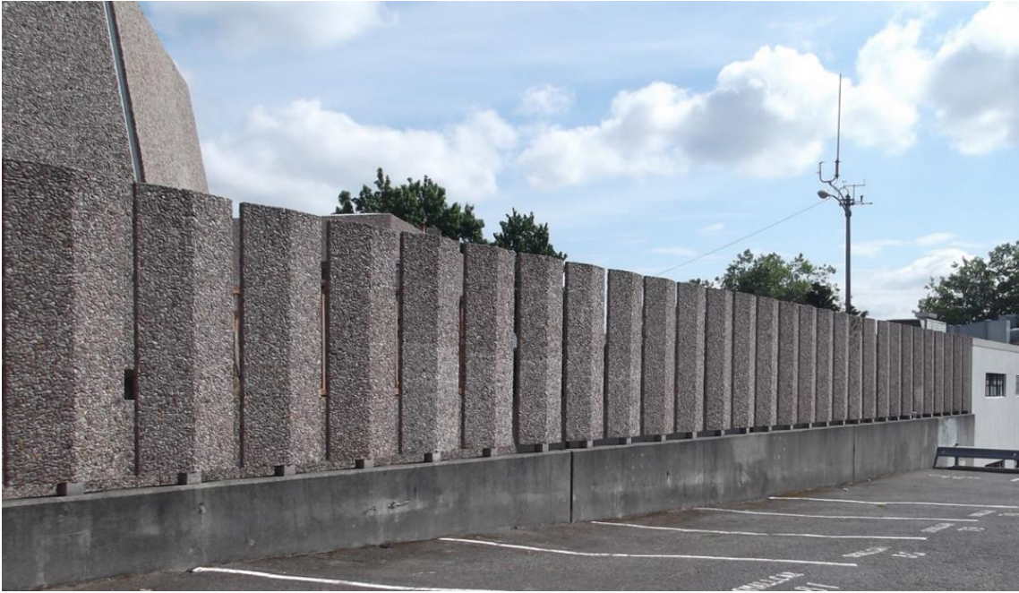
Figure 17: Chevron shaped fence panels. Looking northeast. Photo Date: 2015.
